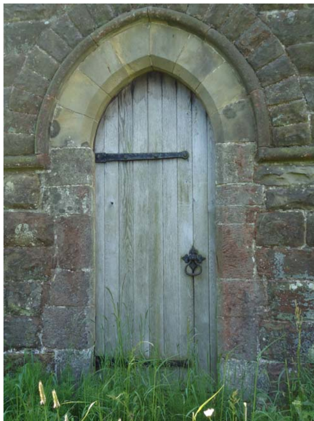
The north door of Reighton church, inside and out.
