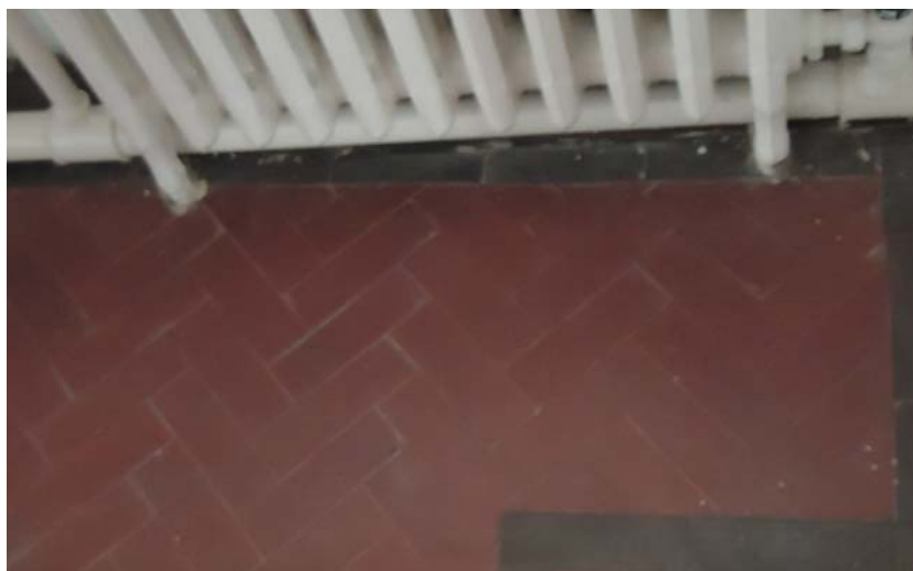
Tiles on the floor of the chancel in Reighton Church
