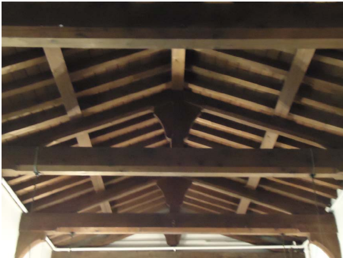
The roof of the nave of Reighton Church
